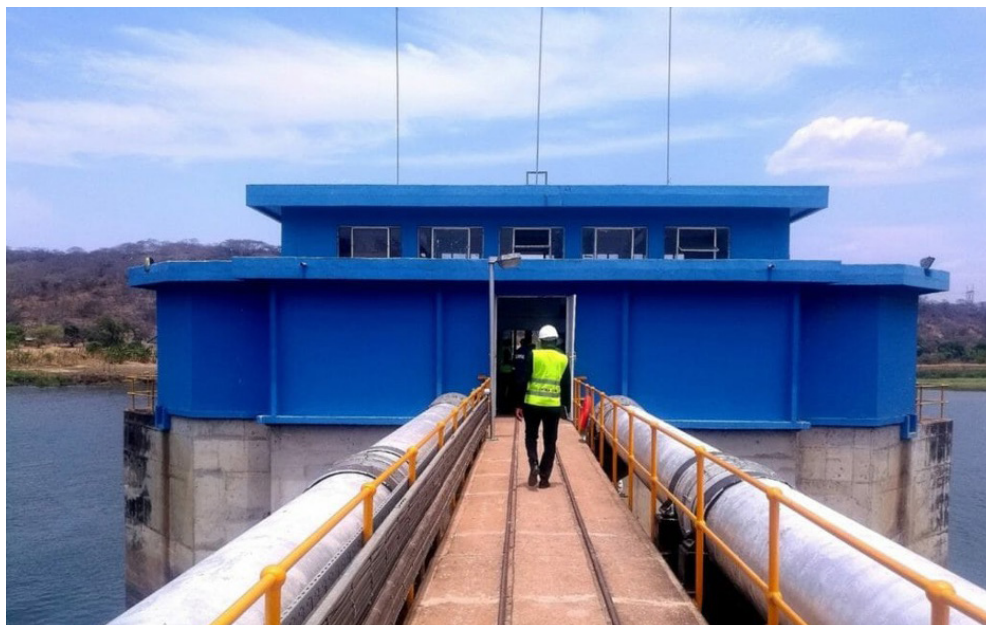
Figure 33 Kafue Water Treatment facility. © Tkach & Chikamba, 2022
